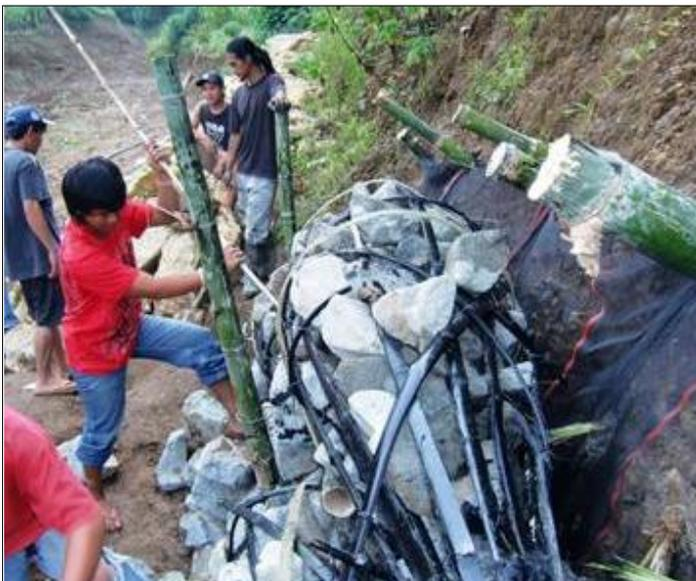
*Reinforcement of a roadside at risk of being eroded during the floor season. The gabion consists of split bamboo.*
